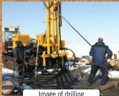
Image of drilling process
